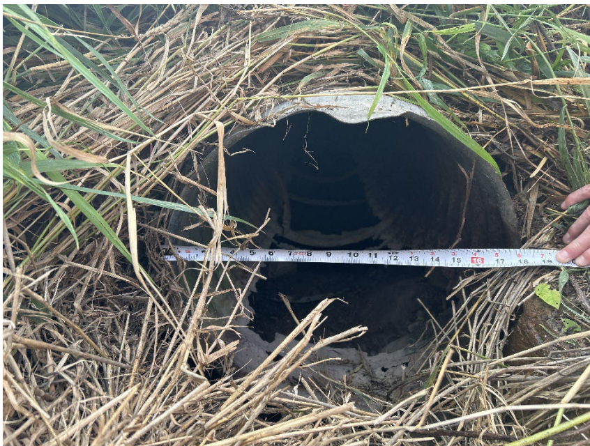
Photo 4 Looking south/downstream through culvert under Lily Lake Road, September 2023.
