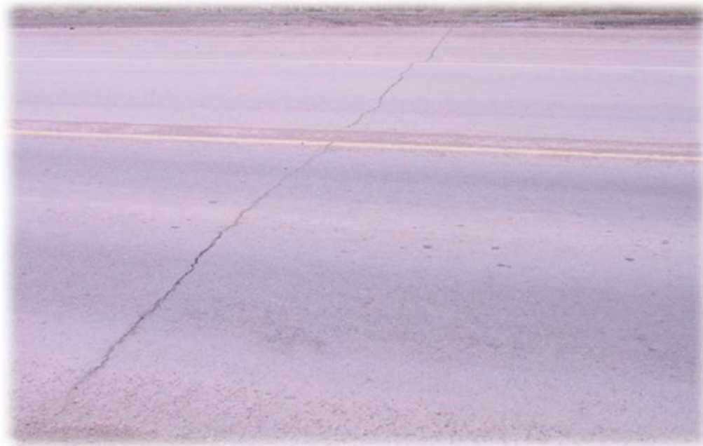
Figure 7: Transverse /Thermal Cracking (Non Structural)
