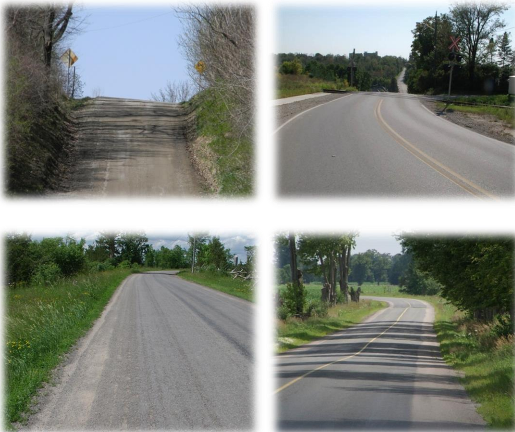
Figure 3-2: Potentially Substandard Vertical and Horizontal Alignment
