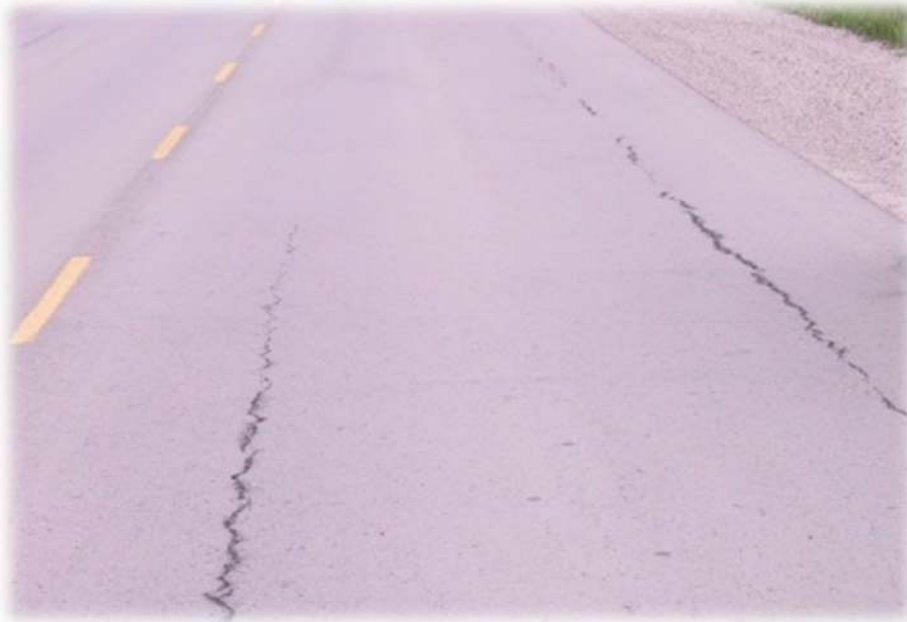
Figure 3: Wheelpath Fatigue Cracking
