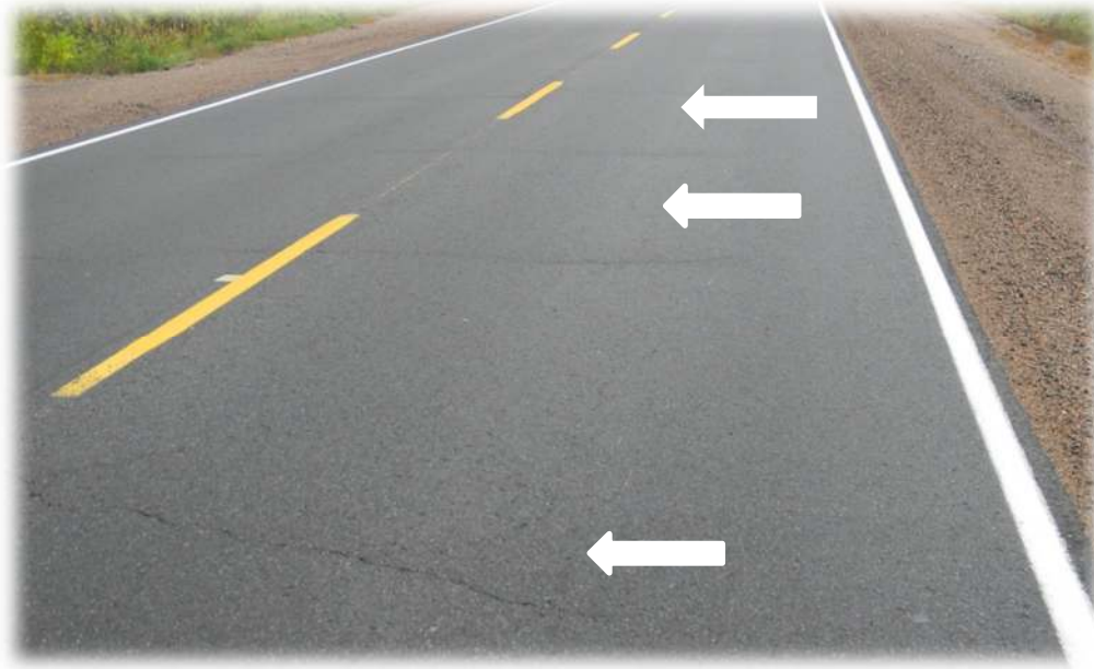
Figure 8: Reflective Transverse Cracking on Newer Pavement
