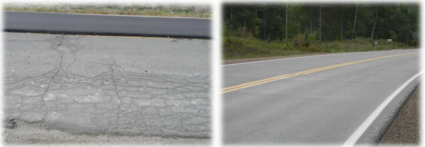
Figure 9: Overlay on Failed Pavement and Resultant Reflective Cracking
